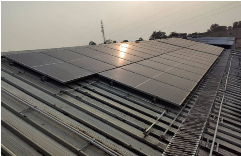
Installed Solar Panels at Mahad Plant with 95 KW capacity
